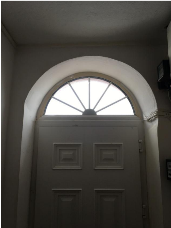
Fig.23; Spoked fan-light over front entrance.
