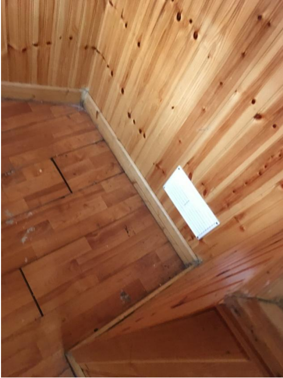
Fig.27; Side room adjacent to Queens Trc; air-vent.
