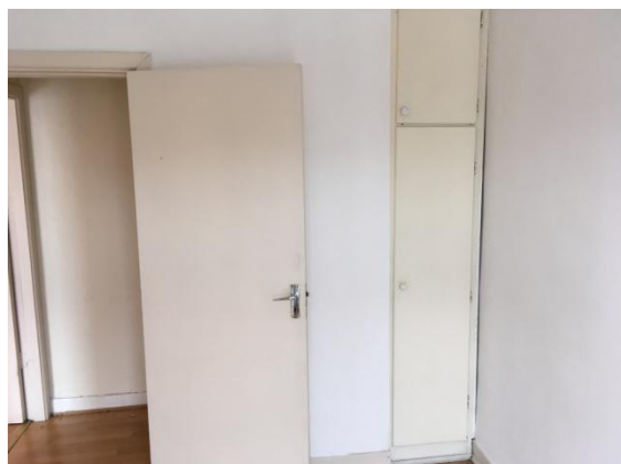
Fig.12; Internal finish at second-floor; flush panel doors
