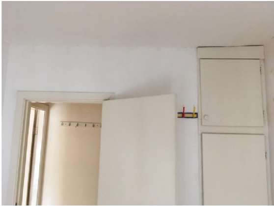
Fig.7; Internal finish at second-floor; flush panel doors.
