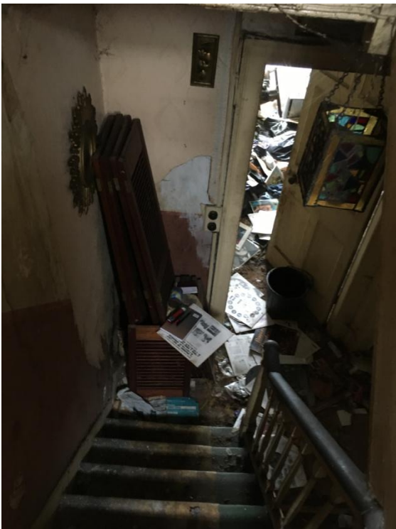
Fig.53; View from return in stairs to first-floor level.
