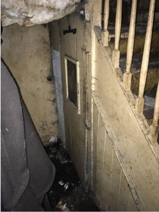
Fig.61; Existing store beneath stairs in entrance hall.
