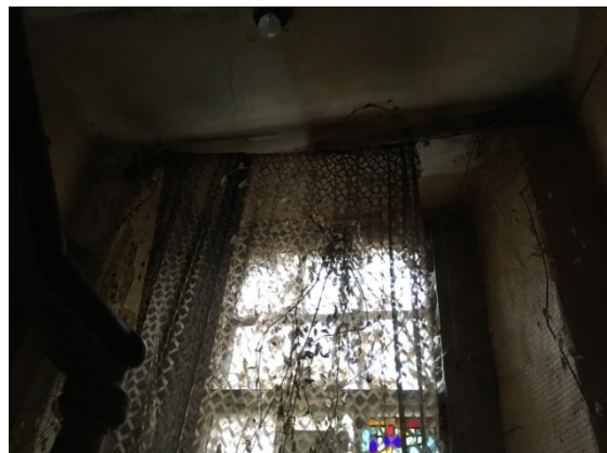
Fig.60; Front window to Thomas Hill; original sliding sash
