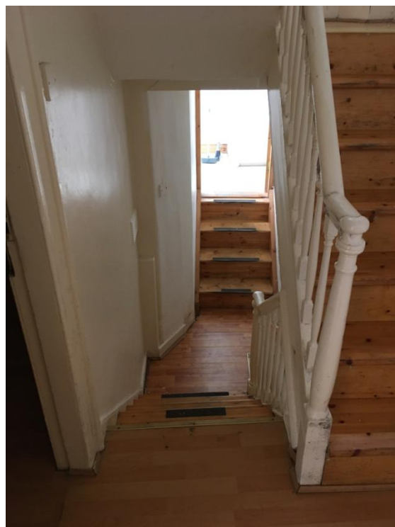
Fig.6; Internal arrangement of stairs at first-floor level.
