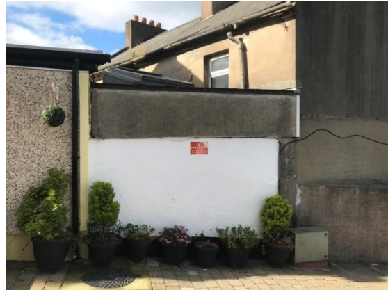
Fig.34; Behind this wall is the first-floor rear extension.
