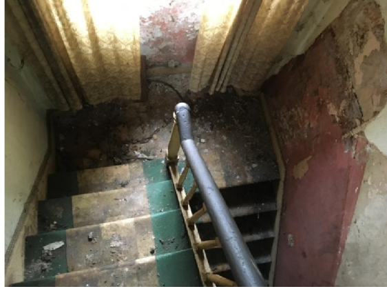
Fig.50; Return in stairs between second & first-floors.
