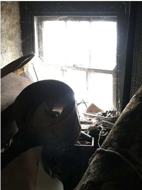
Fig.63; First-floor, rear room; window overlooking yard.
