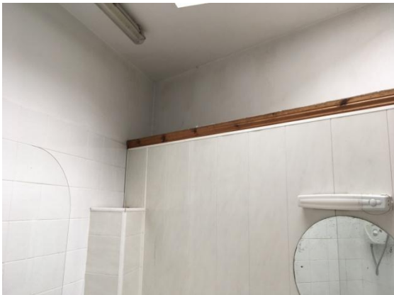
Fig.19; Bathroom at first-floor mezzanine.
