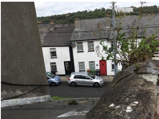
Fig.41; View over single-pitch of side-roof to street.
