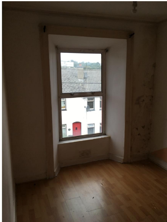
Fig.10; Window to Thomas Hill at first-floor; no shutters.
