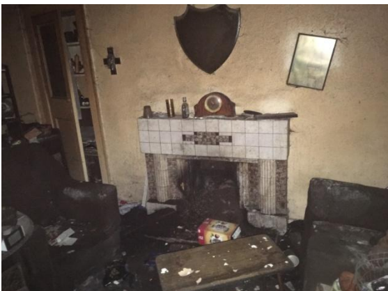
Fig.59; 1950's tiled fireplace in ground-floor room
