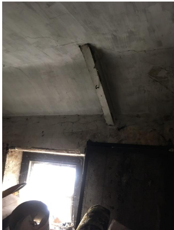
Fig.54; Feature in ceiling at second-floor level.
