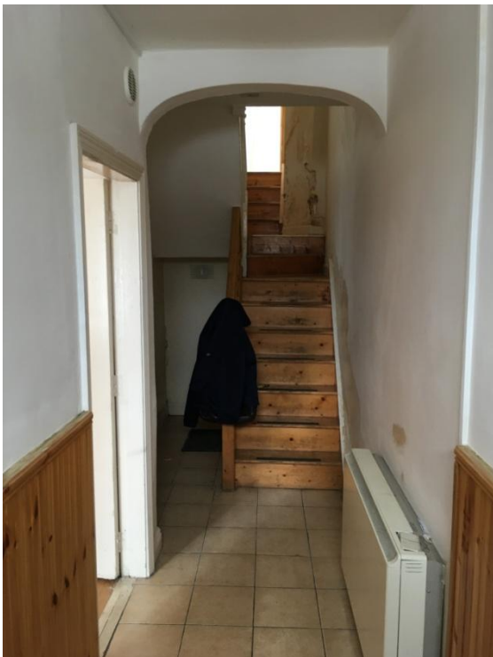
Fig.21; Entrance hallway; minimal detail / character
