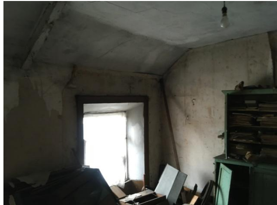
Fig.52; Top (second) floor – rear room; dry and clean.
