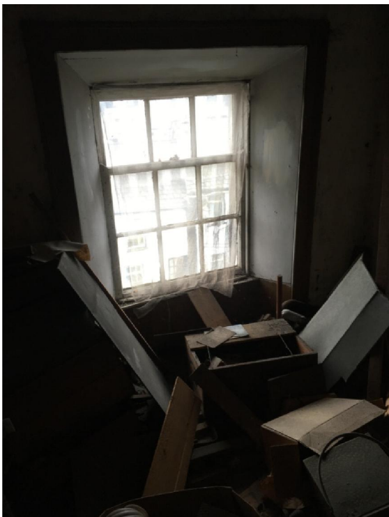
Fig.47; Top (second) floor window on to Thomas Hill.
