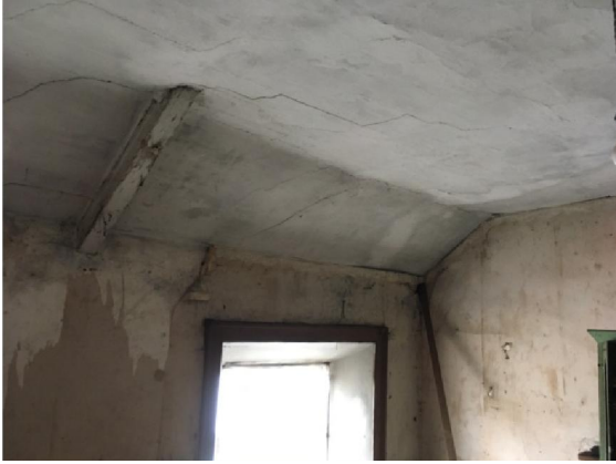
Fig.49; Top (second) floor – rear room; dry and clean.
