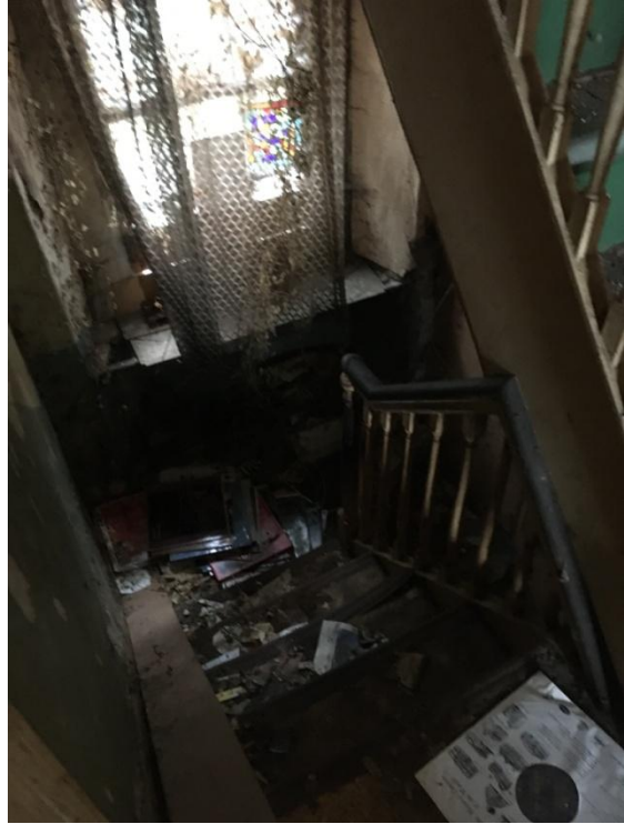
Fig.62; View from first-floor of mezzanine landing.
