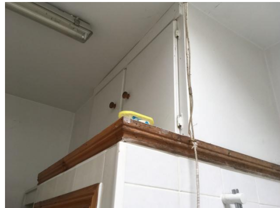
Fig.20; Bathroom at first-floor mezzanine.
