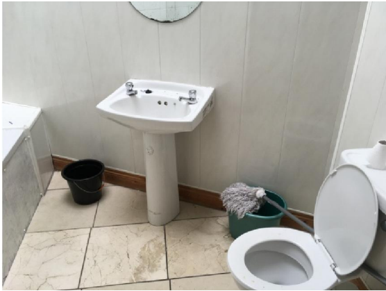
Fig.17; Bathroom at first-floor mezzanine.
