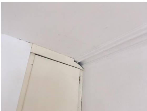
Fig.11; Internal finish at first-floor; arrangement of cupboards against the coving detail suggests sub-division of larger room.
