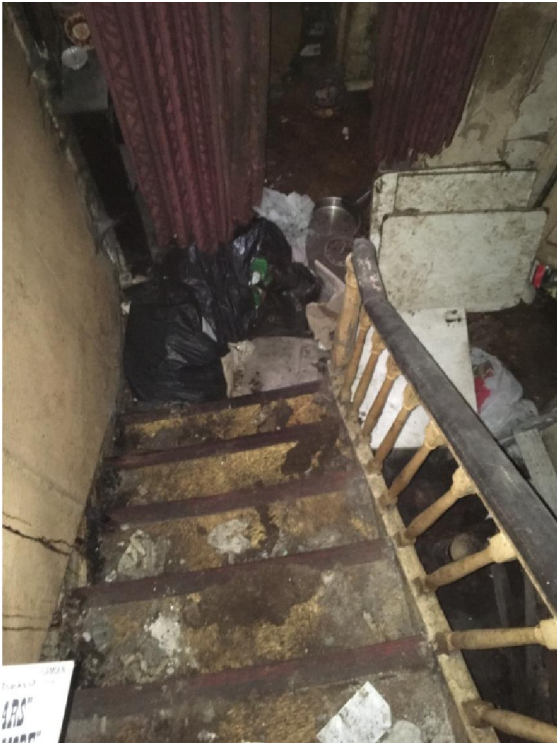
Fig.57; View from landing to ground-floor hallway.
