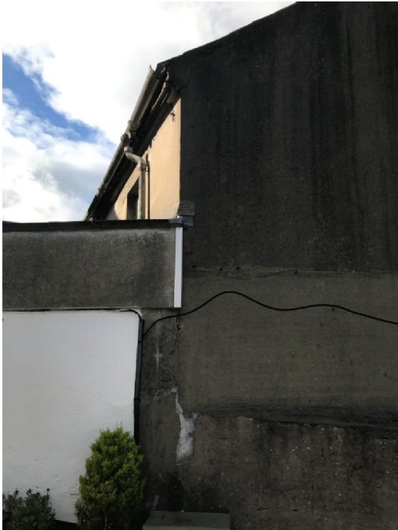
Fig.39; Extension to rear of no.23.
