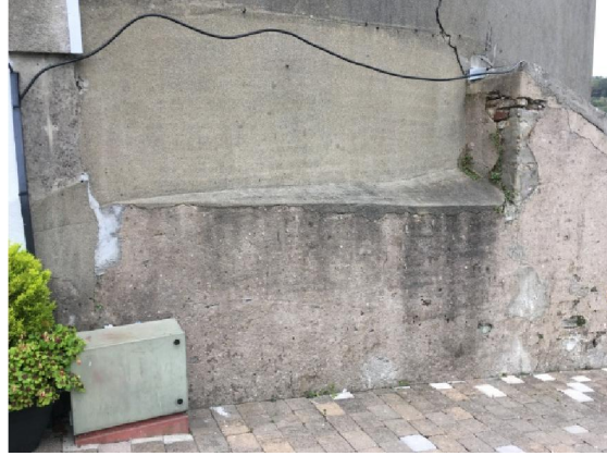
Fig.32; Part of gable-wall of no.23 on to Queens Terrace
