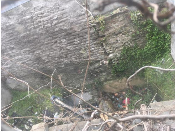
Fig.43; View from top floor into rear garden area.
