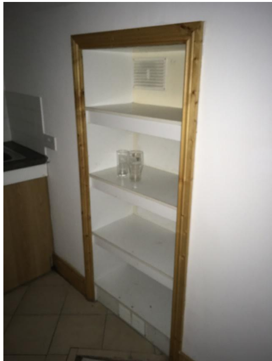
Fig.30; Shelving to rear of no.23; former window ope.
