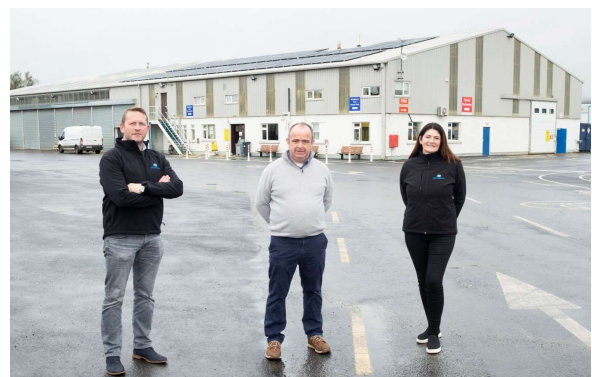
Image: Solar panel installation, Dungarvan Depot
