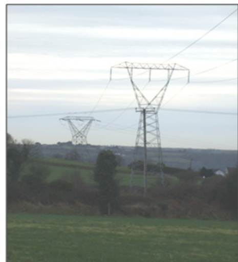
Overhead Power Lines
