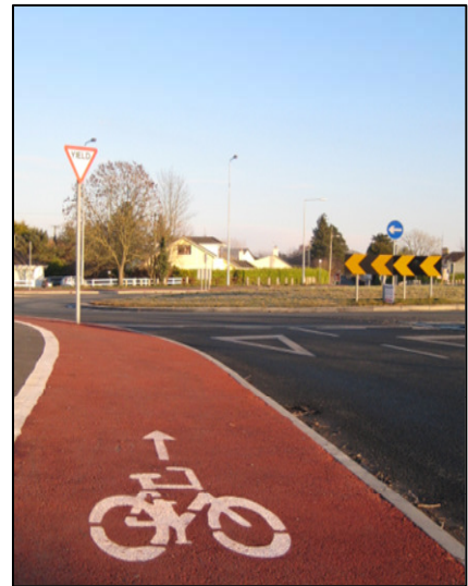
Cyclist Provision at Clonea Road Roundabout
