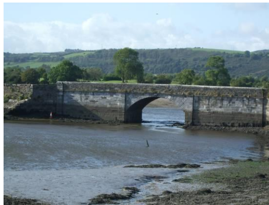
Figure 4. Bridges can provide suitable roosts for bats
