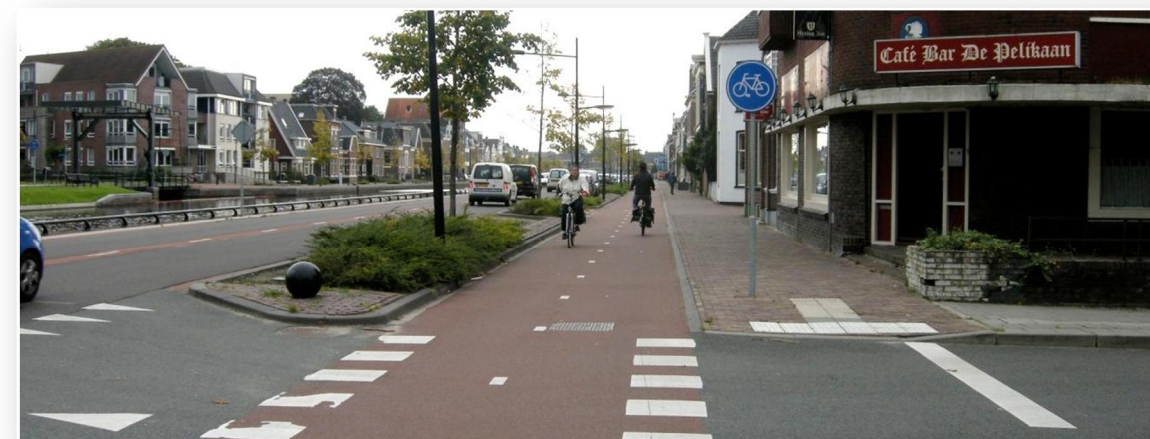
P27 : Dutch Example of a Segregated Two-way Cycle Track in an Urban Environment
