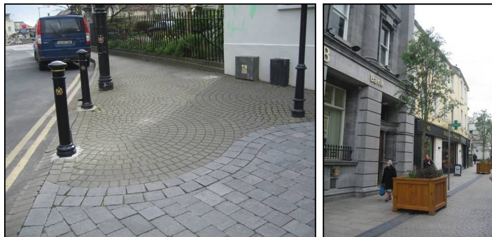
Images 5.17 and 5.18: High Quality Paving and Good Pedestrian Environment
