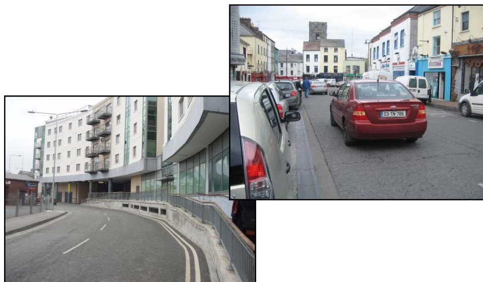
Images 5.19 and 5.20: Poor Pedestrian Environment—Railway Square and Arundel Square
