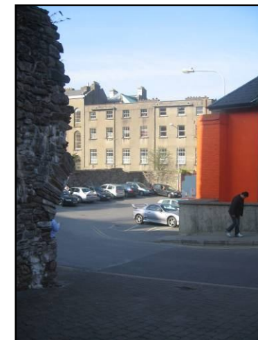
Image 8.6: Extensive buildings onto Georges St that could be incorporated into re-development
