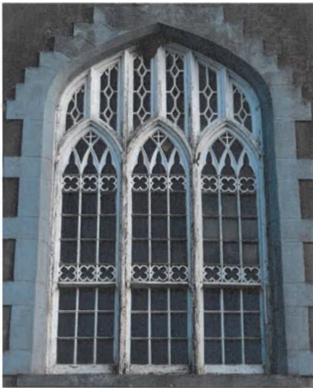
Before works to main frame
