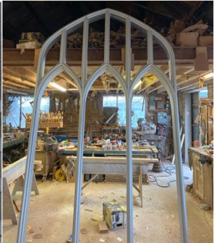
After Frame repaired and painted
