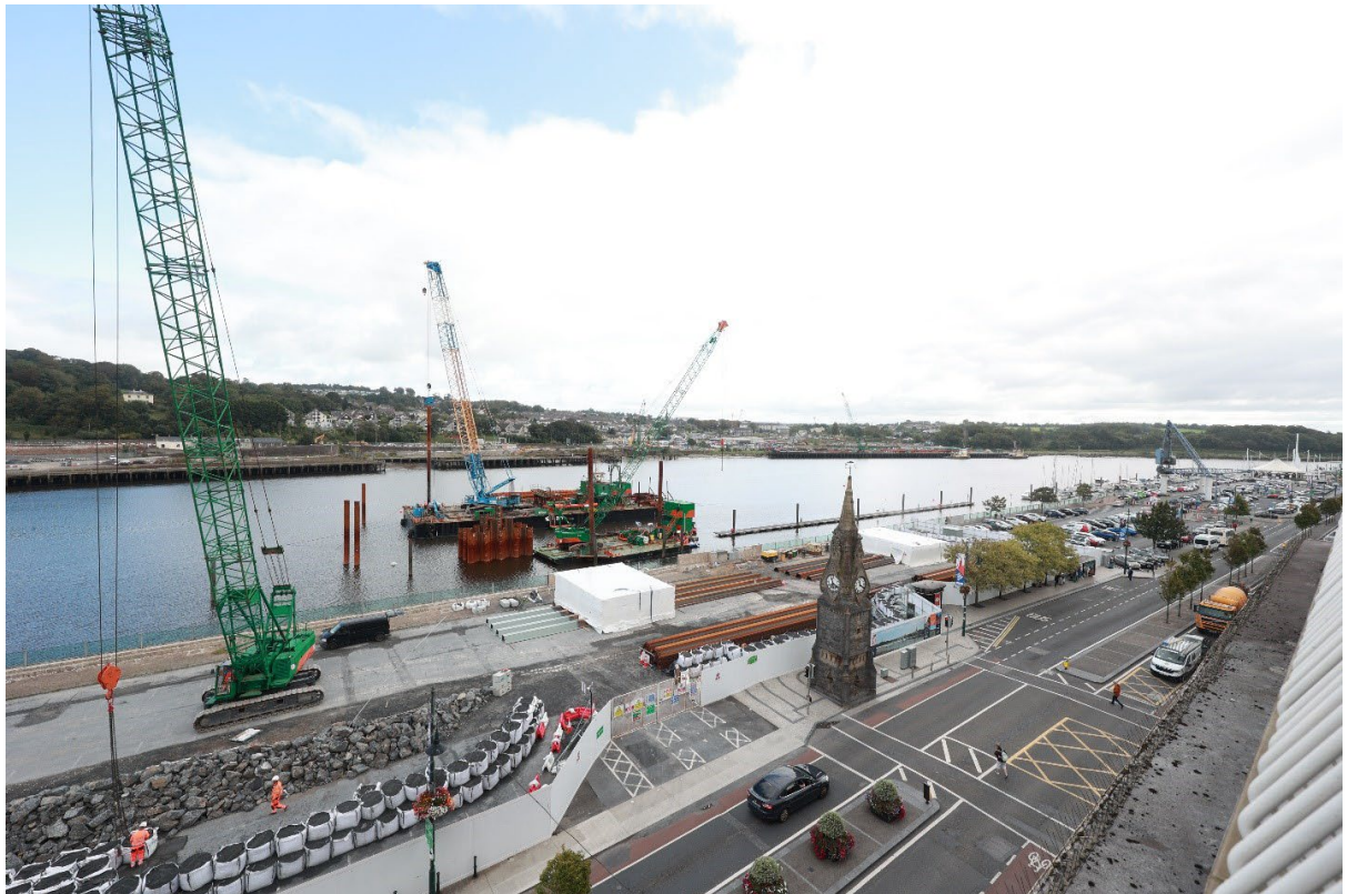
Sustainable Transport Bridge Cofferdam Construction
