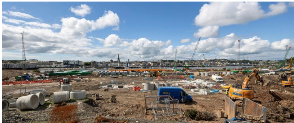
Works progressing at Ferrybank pump station
