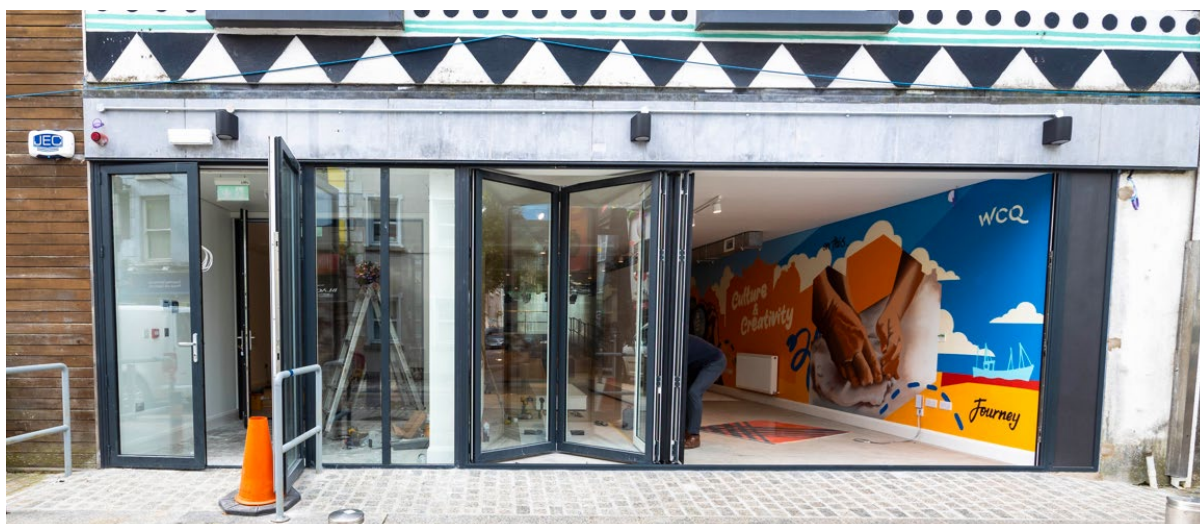
16-18 Barker Place (Project L) – works substantially complete
