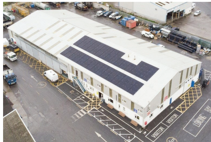
Figure 3. Solar Array on Dungarvan Depot
