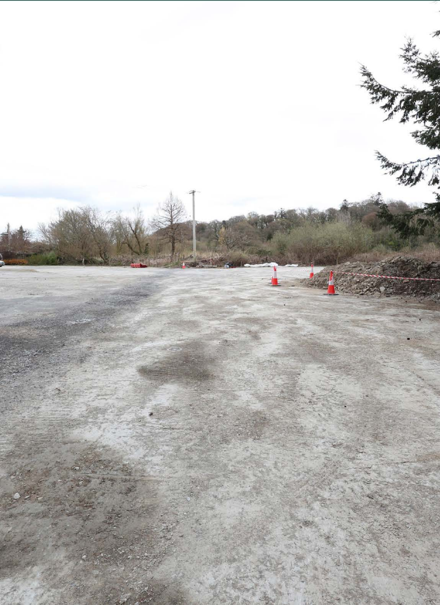
MAIN CARPARK- BEFORE
