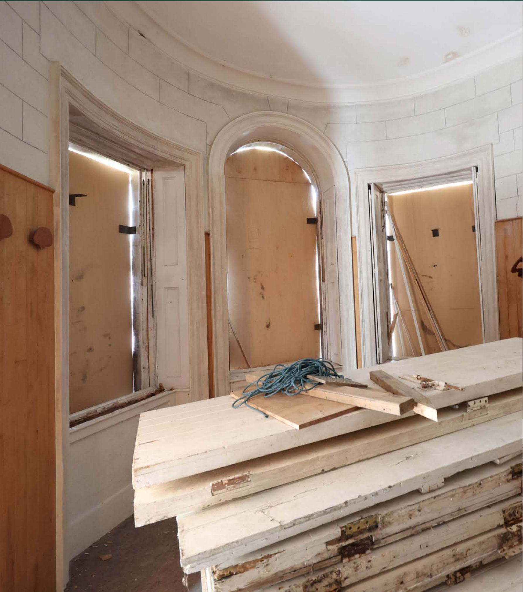
TACK ROOM – BEFORE
