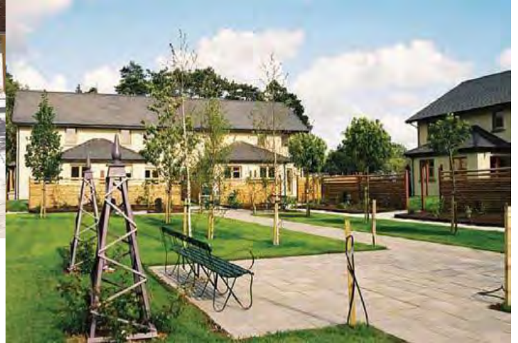
Figure 26: (left) Activity on a shared surface street at Furry Hill, Dun Laoghaire Rathdown County Council. Removing cars and their associated design requirements (kerbs, barriers, markings) signals clearly that this is a street designed for people and allows for relaxed activity by residents (Source, Urban Design Manual 2009).
