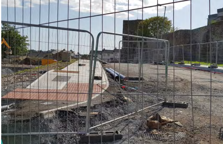
Image 5.10: Brown's Lane road improvements
