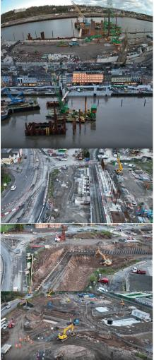
The North Quays main contract works are progressing well. For the Sustainable Transport Bridge the concrete infill stage for the first cofferdam (gridline E) is complete and the process for dewatering the second cofferdams (gridline D) is progressing.
