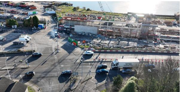
All piling for the Transport Hub building and platforms is now substantially complete. The remaining foundations are nearing completion, and the superstructure is also progressing (rising walls, slabs, supporting walls, etc.). Irish Rail is continuing to install a new rail track to the south of the existing rail track, see below.
