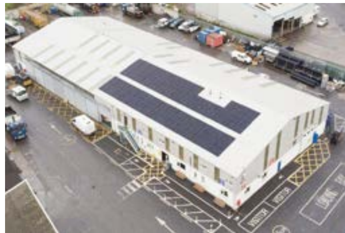
Figure 3. Solar Array on Dungarvan Depot
