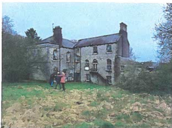
View from interior of site
