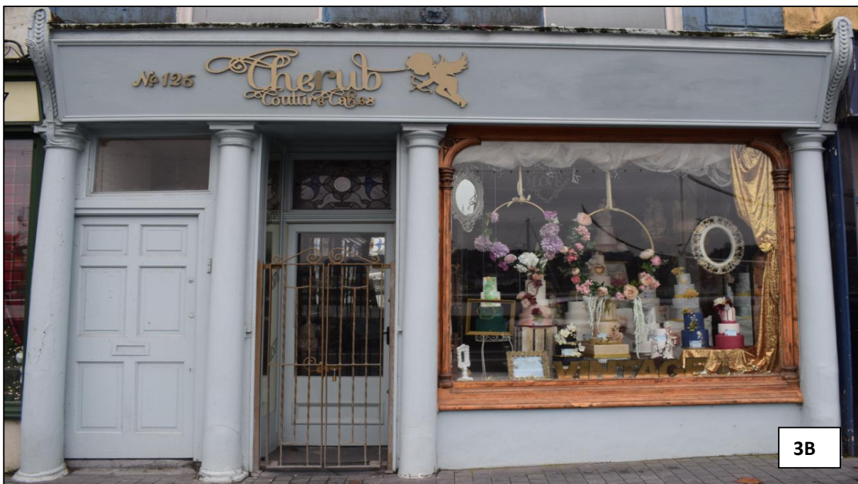
Figure 3 – Upper Floors: Image A depicts brass name plate at entrance door; Image B depicts shopfront which has retained access to upper floors.
