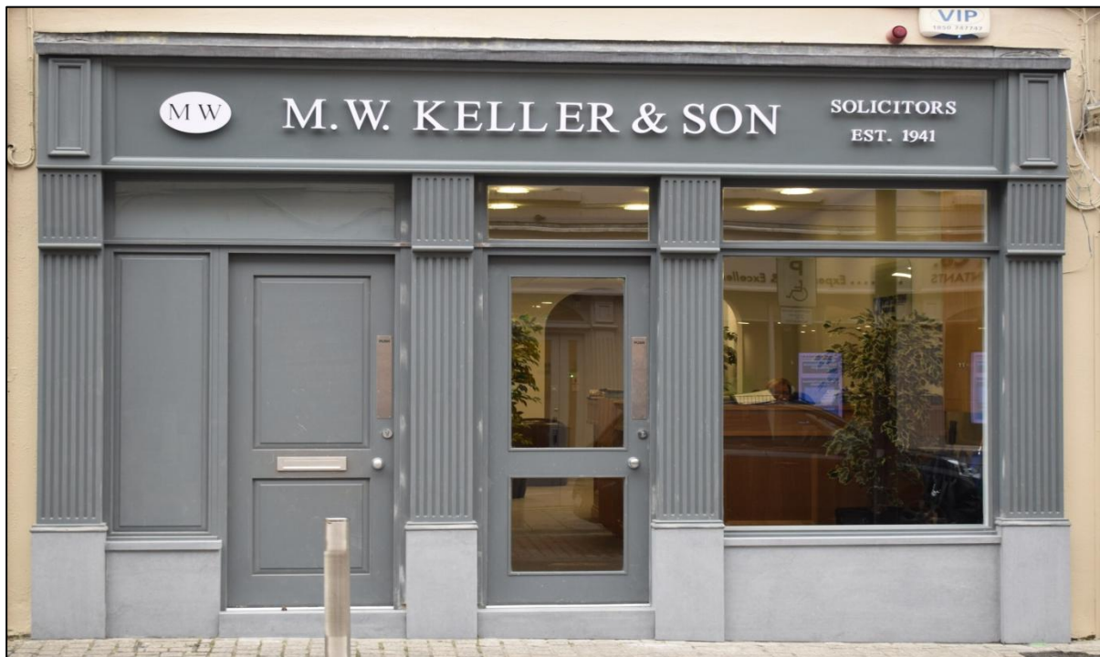
Figure 5 – Upper Floors: depicts a contemporary shopfront which has retained access to upper floors.
