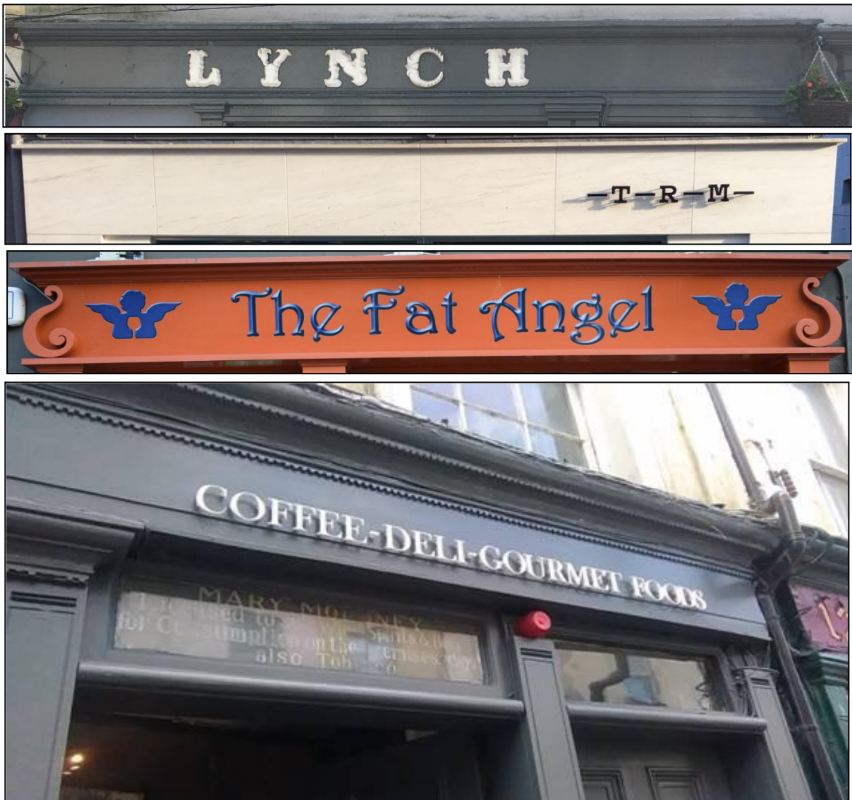
Figure 2 – Fascia Signage: acceptable signage which is in proportion to the fascia depth which is either painted on or consist of individually mounted solid letter on the fascia board.
