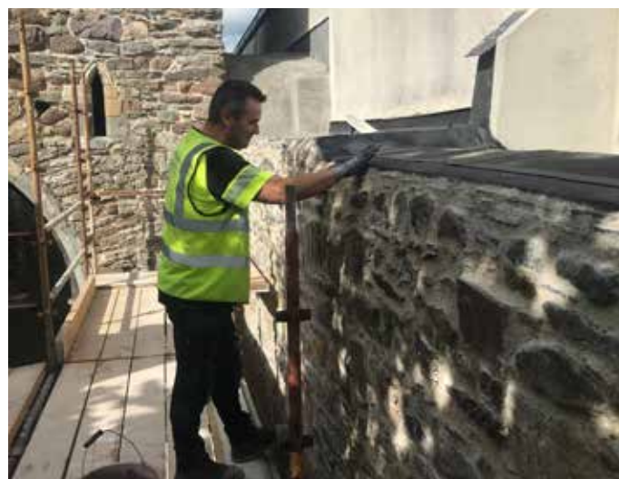
Building conservation works
