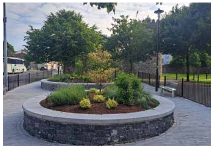
Railway Square improvement works
