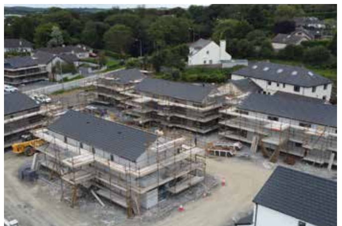
Gort na hInse housing development
