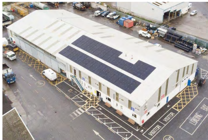
Figure 3. Solar Array on Dungarvan Depot
