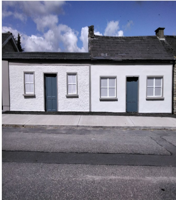
Front Elevation from 8 and 9 Carrick Road, Portlaw after
