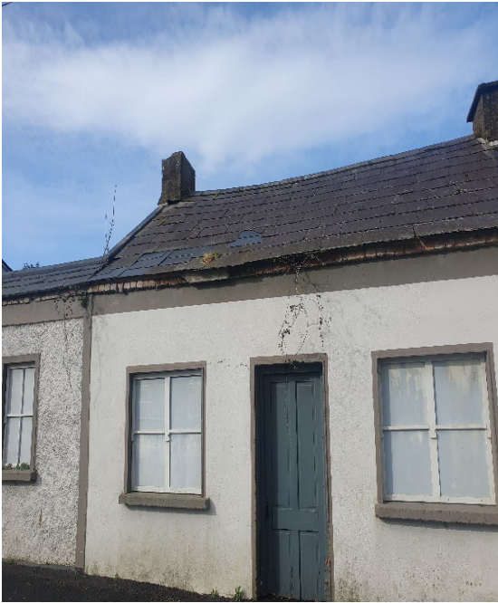
Front Elevation from 8 and 9 Carrick Road, Portlaw before
