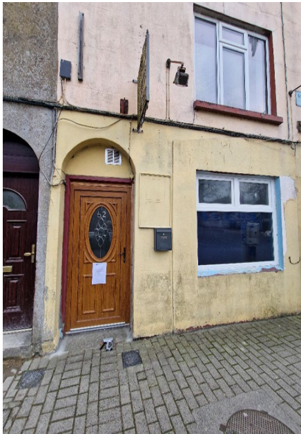
Front Elevation from 52 Manor Street, Before
