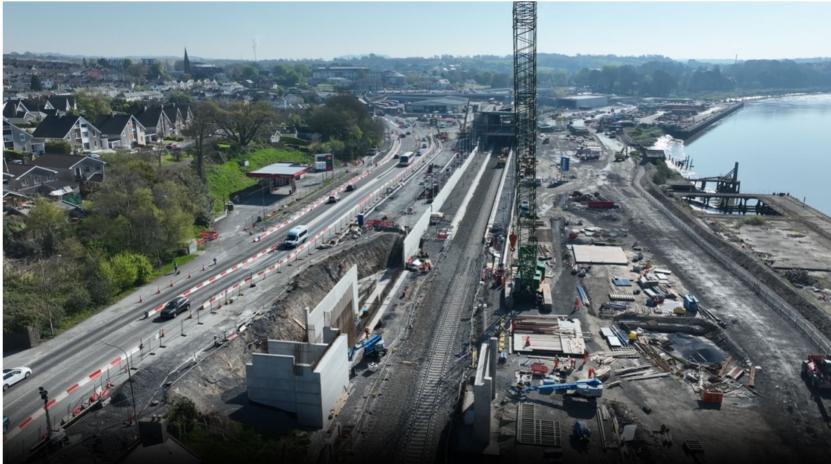
Construction of western footbridge in the foreground that will link directly to the Sustainable Transport Bridge, the platforms and train station are visible beyond
