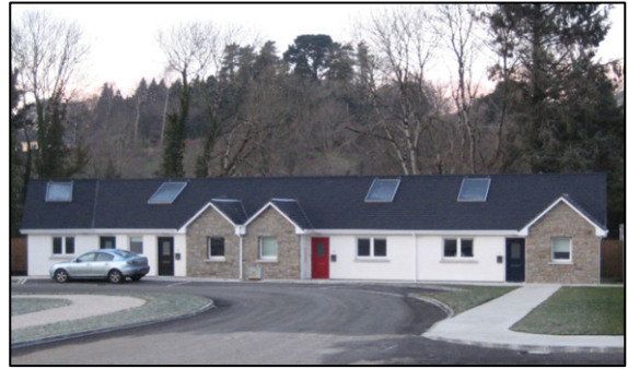
Ballymacarbry Sheltered Housing Development
