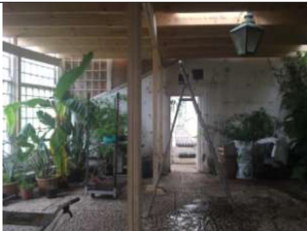
Interior of glasshouse temporary propping of roof – area to be repaired
