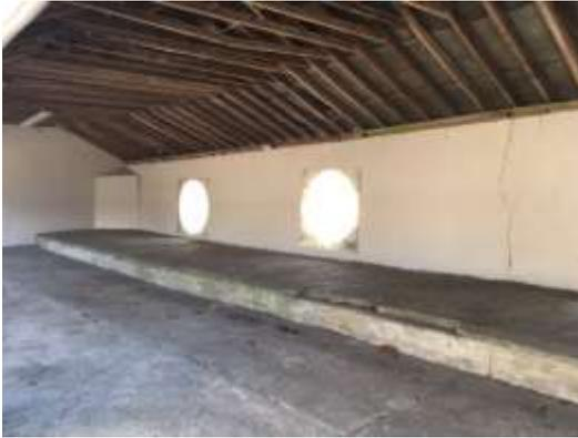
A single storey rubblestone outbuilding with cement rendered walls and pitched roof with natural slate. This is an open shed area which may date back to 19<sup>th</sup> century. Very attractive roof support.
